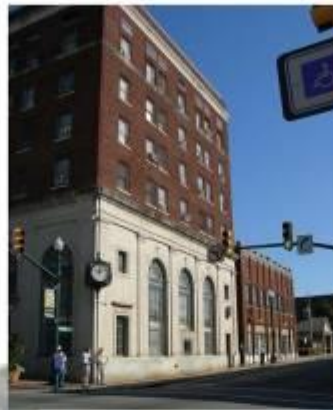
Cabarrus Avenue elevation of the Concord Hotel and the adjacent Bank Building
